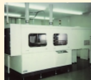
Previously used PCB cleaning tank
