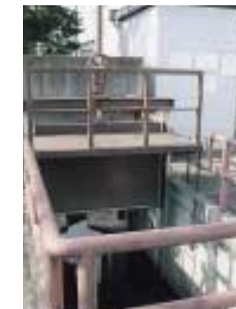
Gate for water channel connected to the outside to prevent harmful chemical substances from leaking out in case of an accident.
