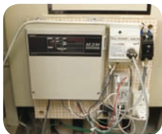
Electricity monitoring sensor terminal installed on power meter
