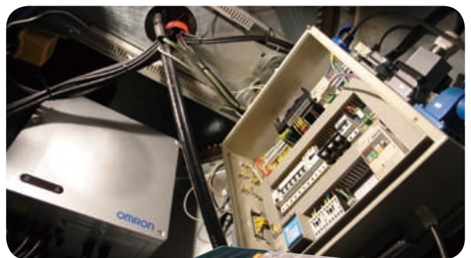
Interior of photovoltaic power system
